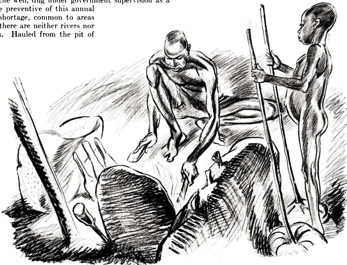
This is a crude, picturesque Nigerian forge. While a boy works goatskin bellows, the blacksmith puts a sharper edge on Sheffield blades or makes simple tools of iron
